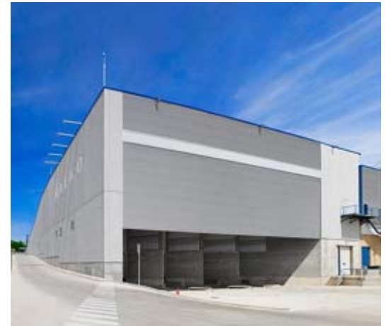
Exterior of current facility
